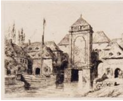
TOURNAI Bridge and Water-Gate
